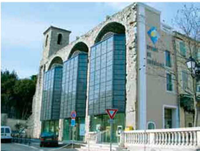
German BIPV Installation: Roofs are not the only building surface where PV can be installed.
